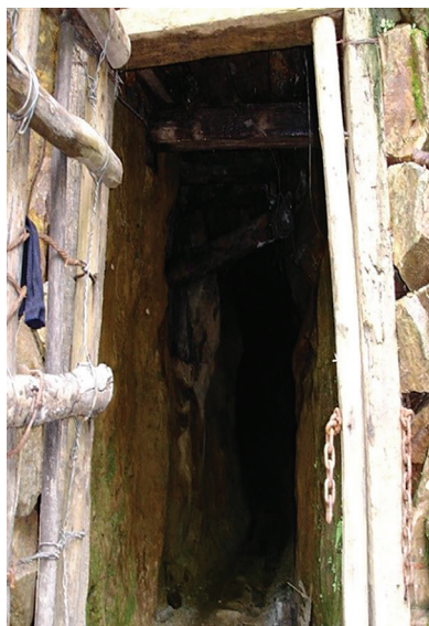
Figure 1. Tunneling Process in Small Scale Gold Mining.
