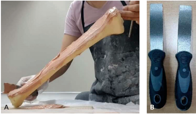
Figure 4. Application of Epoxy Structural Adhesive just enough to cover the surface or approximately 1 mm thick (A) using a clean 1-inch scraper (B).
