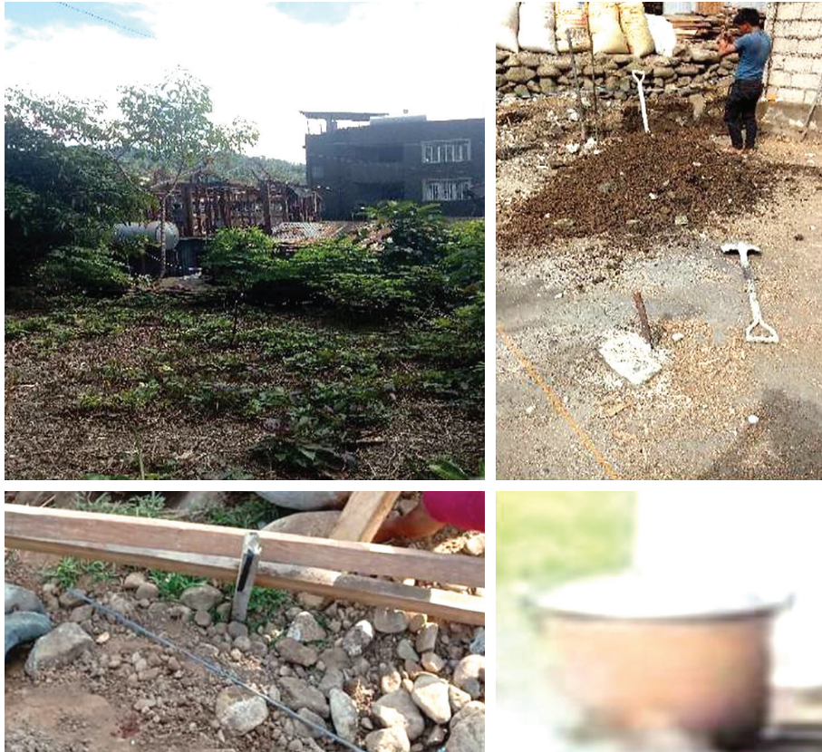
Figure 2. Stages in house construction.
